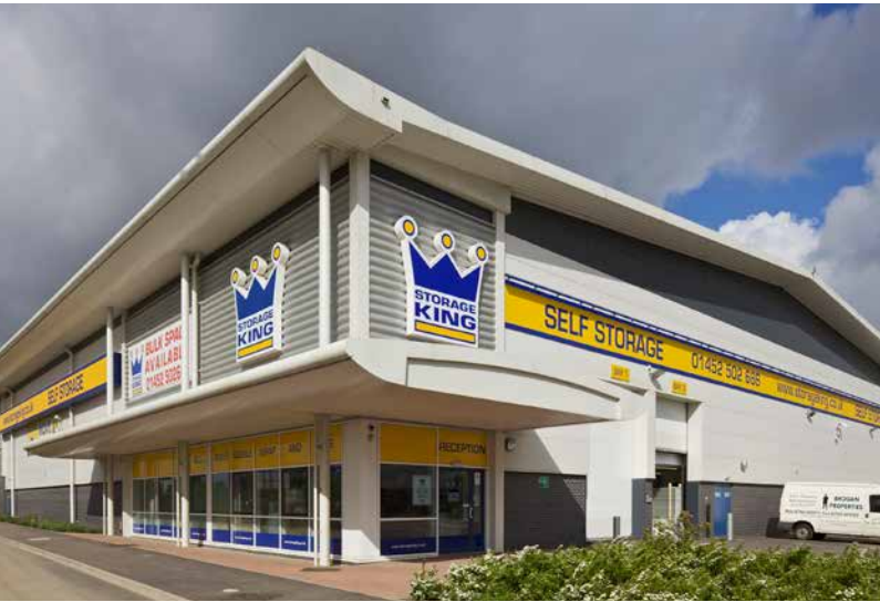
Storage King in Gloucester, England
