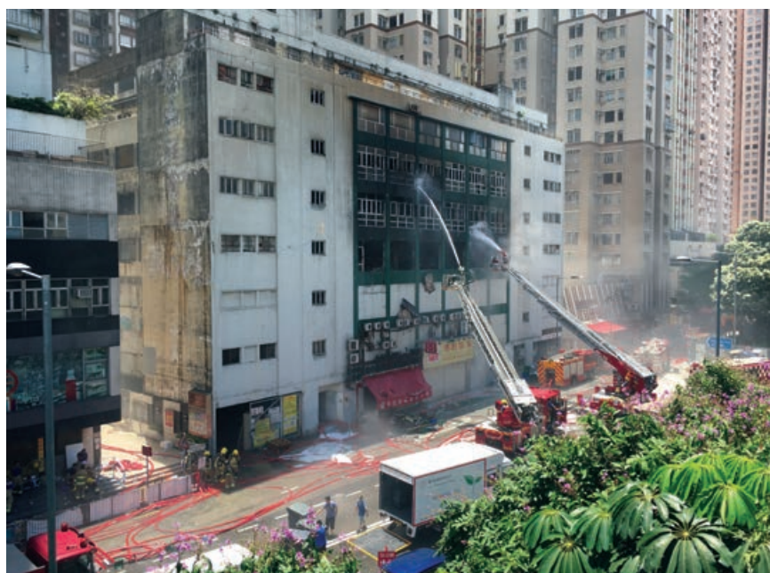
The fireman continue to put out the Ngau Tau Kok fire on June 24 2016
